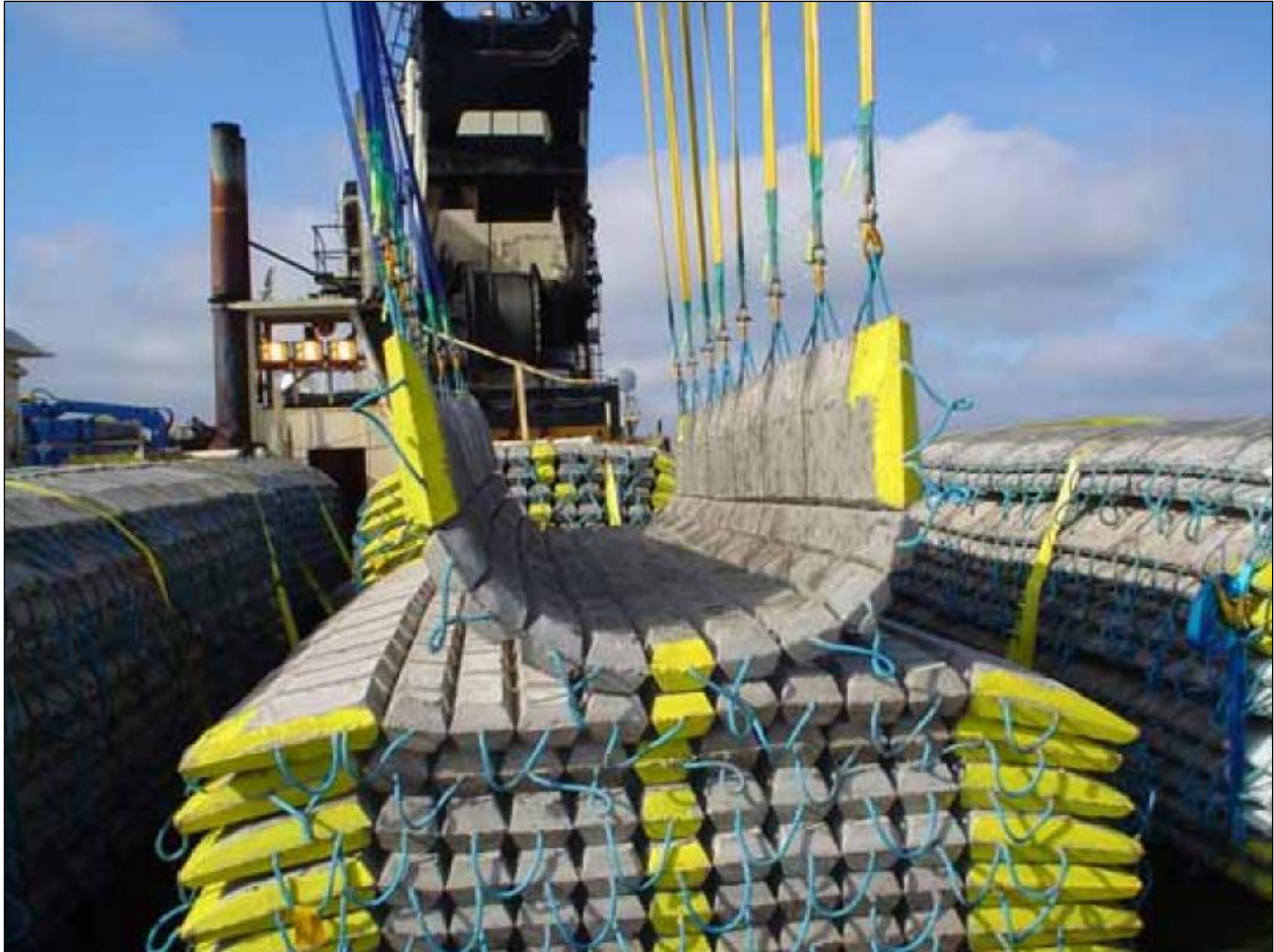
Figure 2-7. Typical Articulated Concrete Mats
